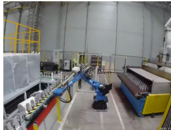
Loader/Unloader Robotic System Status: Live February 2020, Turkey
