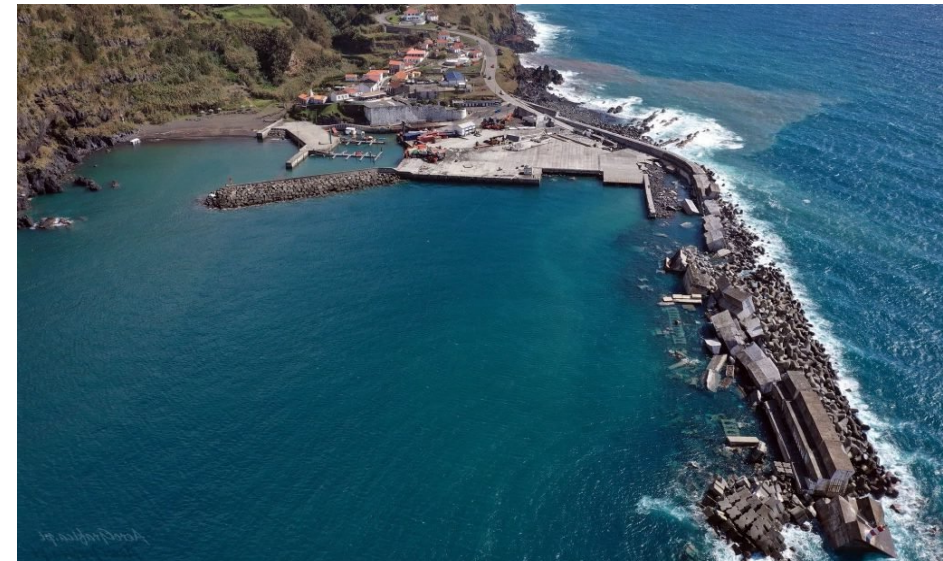
Destroyed breakwater in Flores, Azores.
