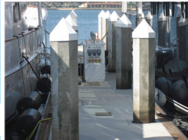
Figure 7.2: Example of insufficient dock width
