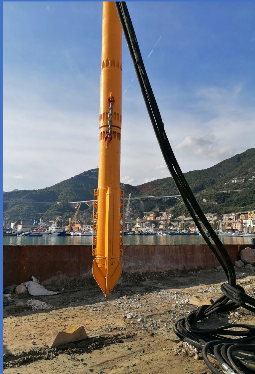
TEST FIELD VIBRO-REPLACEMENT AT THE SALERNO PORT
