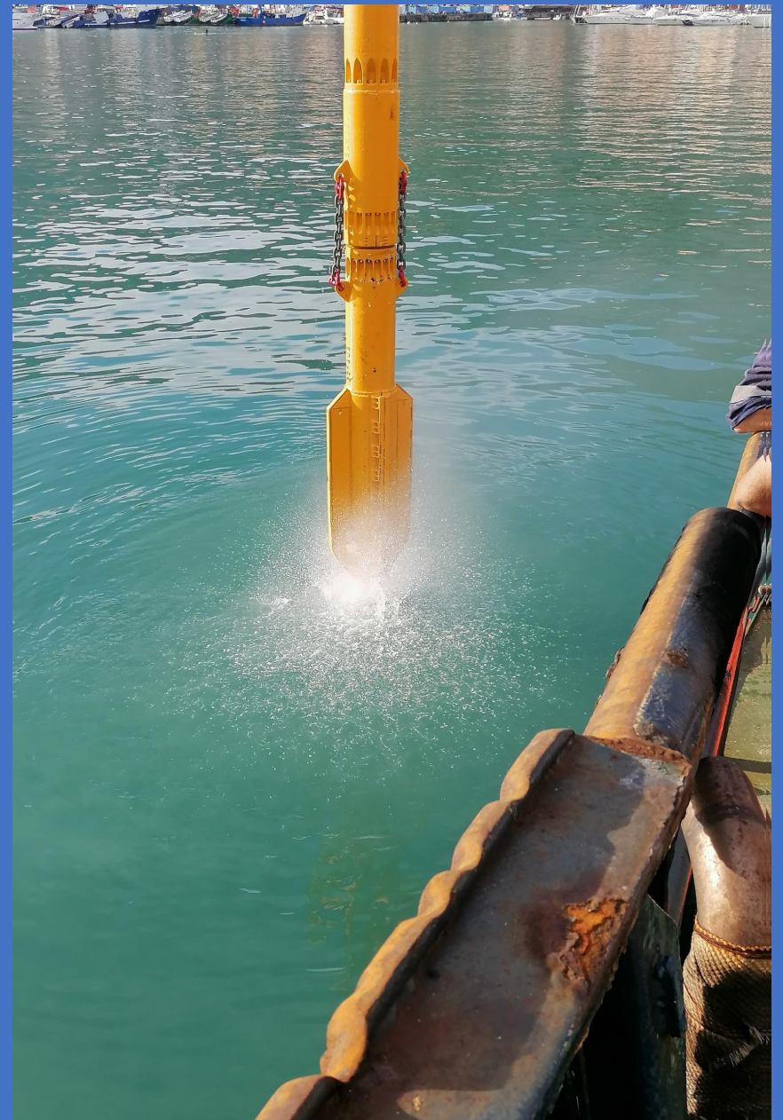
TEST FIELD VIBRO-REPLACEMENT AT THE SALERNO PORT
