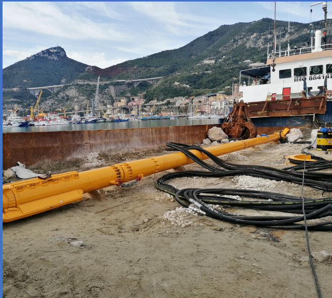
TEST FIELD VIBRO-REPLACEMENT AT THE SALERNO PORT
