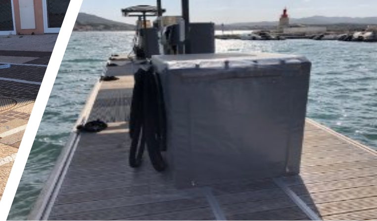
INSTALLATION OF SEWAGE AND BILGE WATER PUMPS
