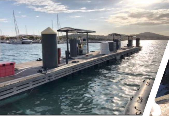
FUELLING SERVICE STATION
