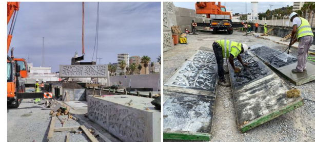
Figure 8.10: Concrete blocks with bio-enhancing admix and texturing for marina application (photo by EConcrete Tech LTD)
